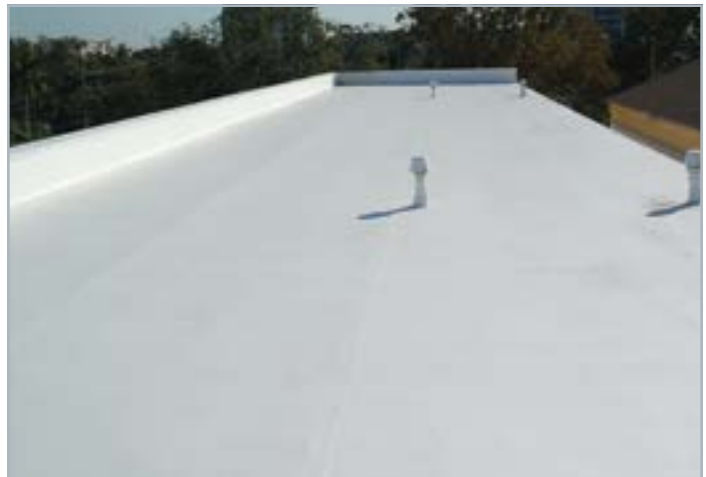
4. Apply ERSystems Polyurethane 300 system or Acrylic 1000 Plus after prep and patching.
