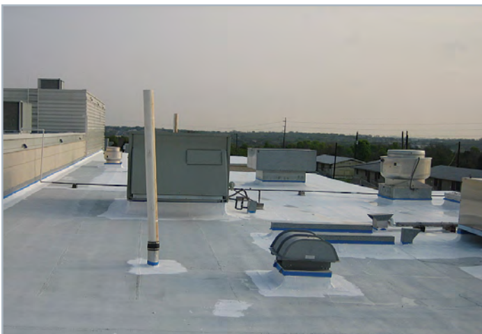
3. Apply ERSystems Acrylic Asphalt Primer/Polyurethane 300 Aromatic Base Coat at recommended rate.
