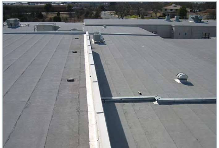
2. SEAL AND REINFORCE around penetrations and flashings.
