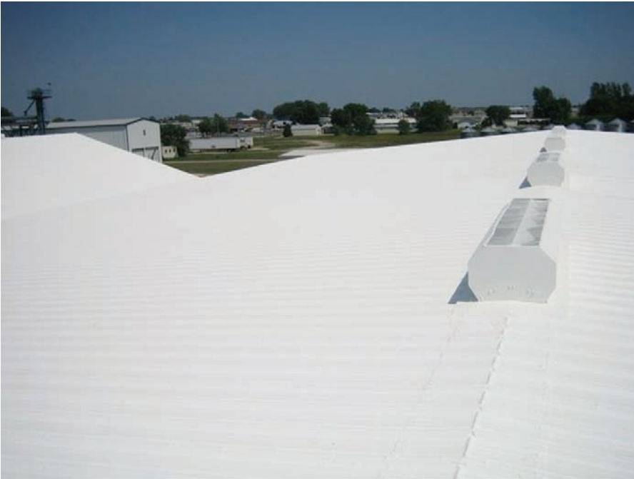
It has become widely accepted in the roofing industry that field-applied white reflective coatings can lower roof surface temperature and provide energy savings.
