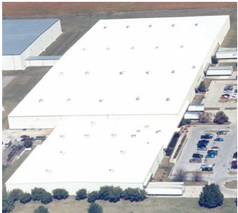
When a coating is light in color, it also can provide a cooling effect to a roof surface. Photos courtesy of ERSystems Inc., Rockford, Minn.
