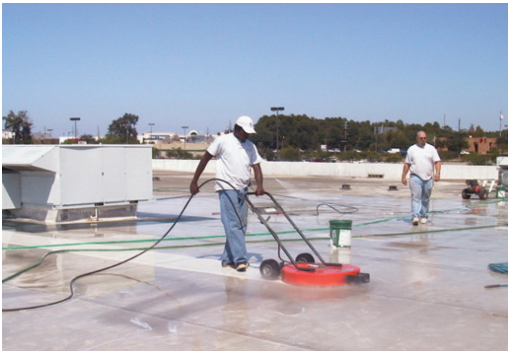
Power washing of a PVC single-ply roof membrane prior to application of coating. All photos courtesy of ERSystems Inc.
