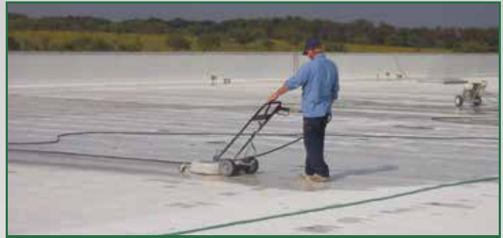
Power wash, removing dirt and debris.
