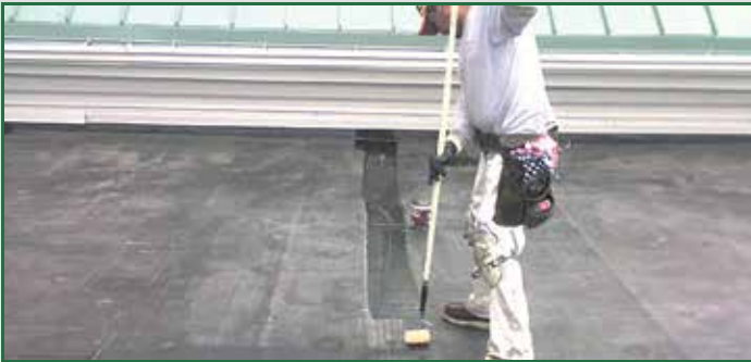
Prime seams, preparing for Fabric Faced Butyl Tape .
