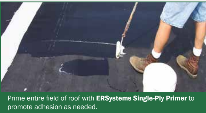
Prime seams, preparing for Fabric Faced Butyl Tape .
