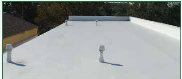
Apply 2 coats of ERSystems Acrylic 1000/SW or Polyurethane 300 Finish Coat . OR 1 coat of OneStep after Fabric Faced Butyl Tape .
