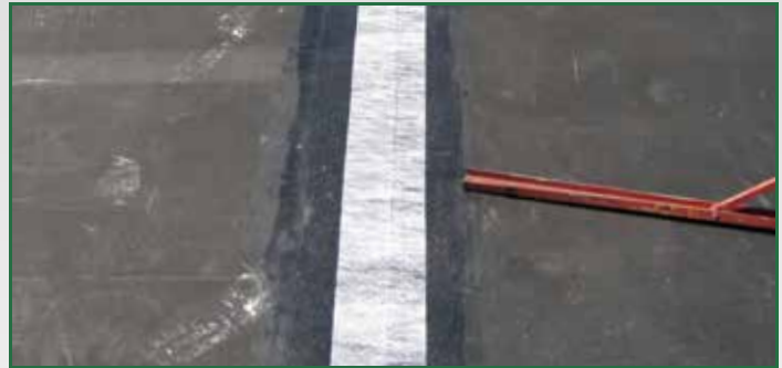
Apply Fabric Faced Butyl Tape to all seams.
