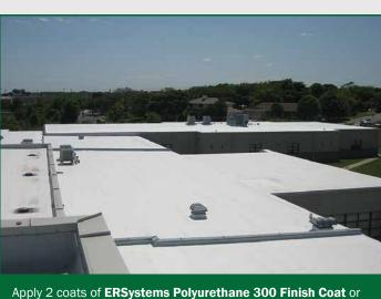
Backroll any vertical surfaces (parapets, walls, etc.).
