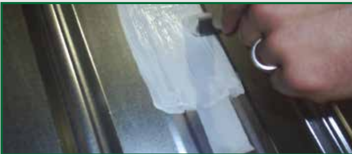
Step 5: Apply second layer of coating over polyester fabric. Let cure for 2-3 days.
