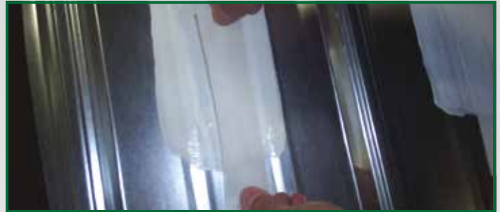
Step 4: Apply polyester fabric into first layer of coating.
