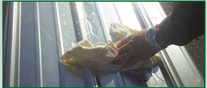
Step 2: Wash substrate and allow to dry.
